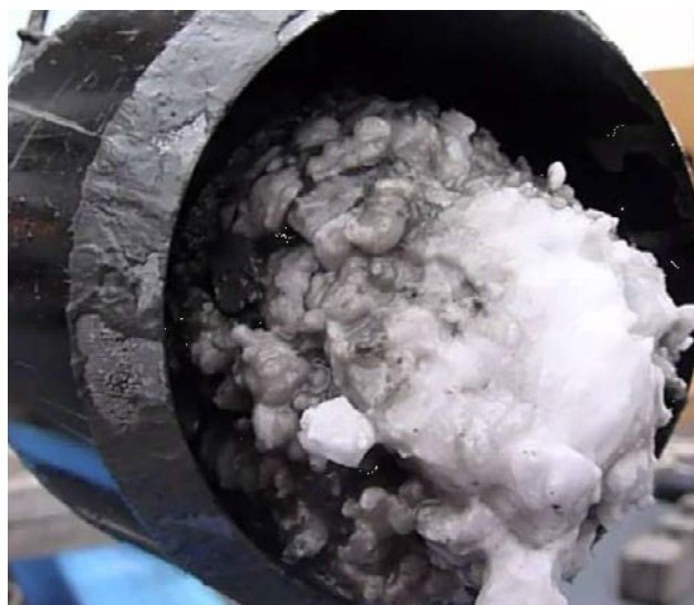
In particular, when a pipeline is idle for a longer time at low temperatures, hydrate plugs can form, similar to the methane hydrate core shown here.
