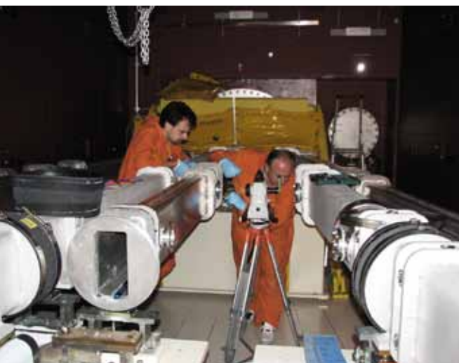
Figure 1: Members of the neutron optics group align a new neutron guide element in the neutron guide tunnel.
