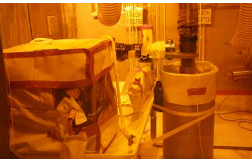
Figure 1: Shearing of the old NEPOMUC experimental tube in the hot cell facility.
