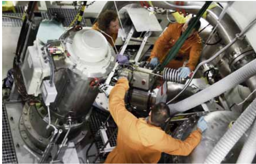
Figure 3: Maintenance work in the primary cooling circuit room.
