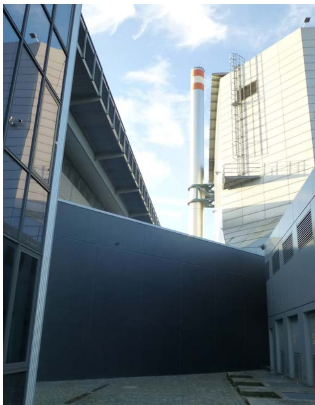
Figure 8: Exterior view of the new connecting building from the north side.
