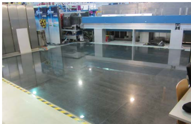
Figure 13: The finished new granite floor for instrument KOMPASS.
